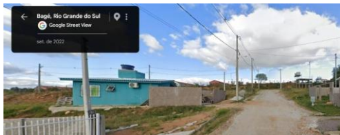
Rua A, Loteamento Oswaldo Betemps — Street View, set/2022
