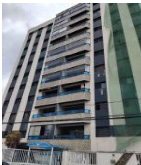
Fachada Cond. San Marino
