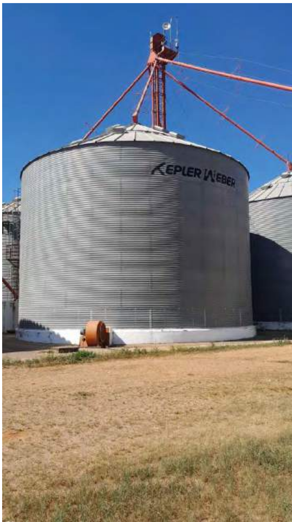
28 - Silo Kepler Weber
