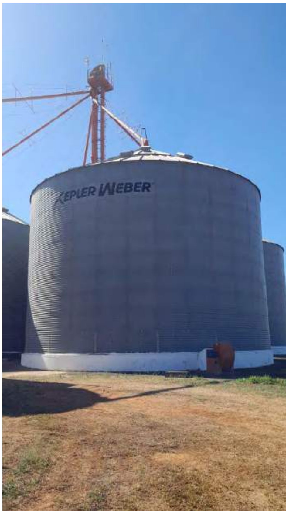
33 - Silo Kepler Weber
