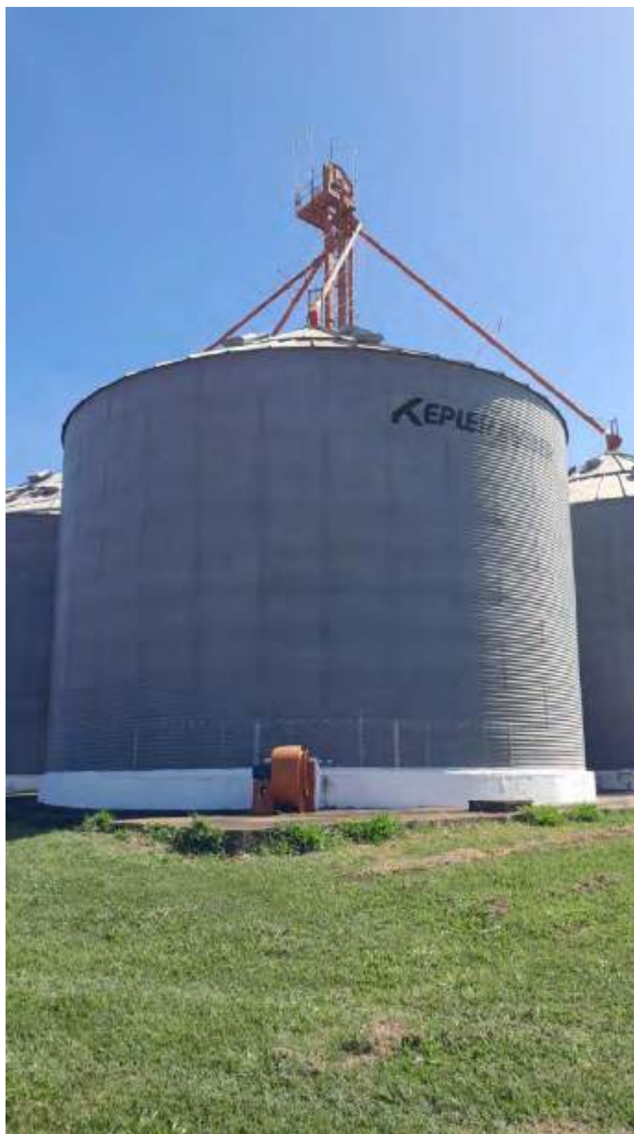
38 - Silo Kepler Weber
