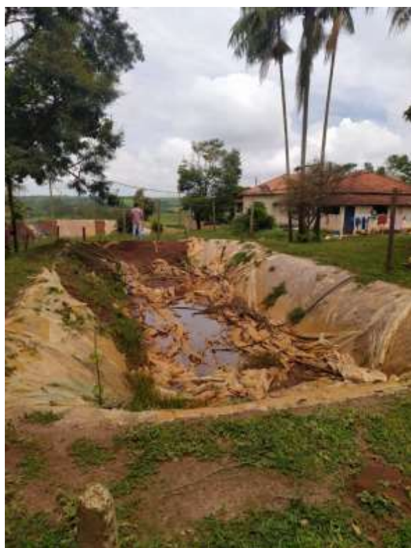
Figura 26- AÇUDE 1 ( A= 116,30 \text{ m}^2 )
